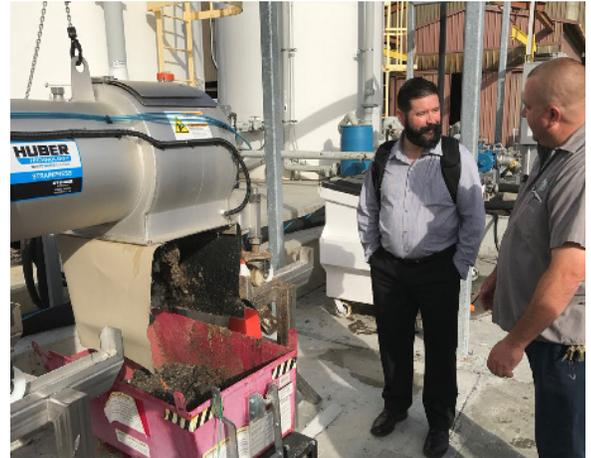
Non-digestible debris was showing up downstream of the strainer which isn’t acceptable if the FOG system is expected to work efficiently. The stream must be cleaned out ahead of reaching the digester because it takes up valuable space, and it also has the potential it has to cause damage.
