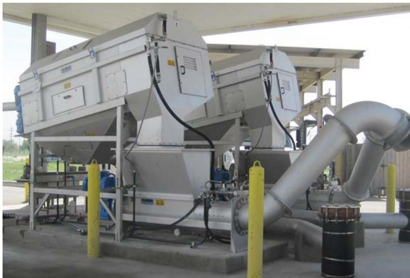
The “hybrid” implementation of Ro 3 and RoFAS units that SAWS now has works well to separate large solids and grit from the septage that passes through the station. There are back-up units for both the Ro 3 and RoFAS on stand-by so
