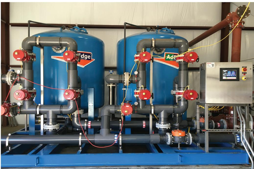
AdEdge Water Technologies, LLC provided four 72-inch carbon steel vessels with AD26 oxidation/filtration media.
