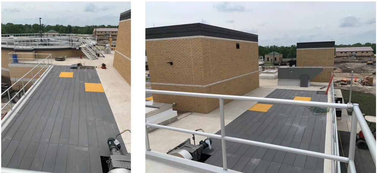
Figure 10: AquaPrime filters with removable fiberglass covers
